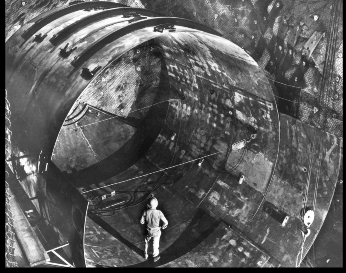
Raymond Davis of Brookhaven National Laboratory constructed a <u>neutrino</u> detector 1.6 km underground in the Homestake Gold Mine in Lead, South Dakota. The detector consists of a 378,000 liter tank of perchloroethylene, which is further isolated by being submerged in water. Theoretical expections were about one neutrino-chlorine interaction per day, but the measured solar neutrino events were about a third of that, raising serious questions about the abundance of solar neutrinos
